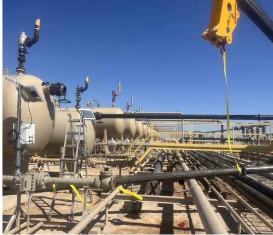
Equipment Construction at Central Facilities
